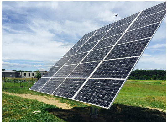
AllEarth Series-24 Solar Tracker, 24 285 W SolarWorld modules, Fronius Primo 7.6 kW inverter, 6.84 kW DC
